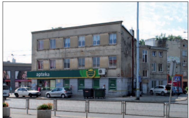
entrance to the Umschlagplatz compound. Genewein took his picture from inside the enclosure. Right: The building stands virtually unchanged at the junction of Zgierska and Limanowskiego.
