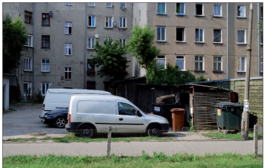
The building at what is today No. 86 Wolska Polskiego survives virtually unchanged.
